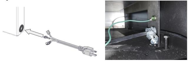
4. Connect the wiring for all components as shown. To connect the ground, it may be necessary to separate the ground wire from the cord by gently pulling the cables.
